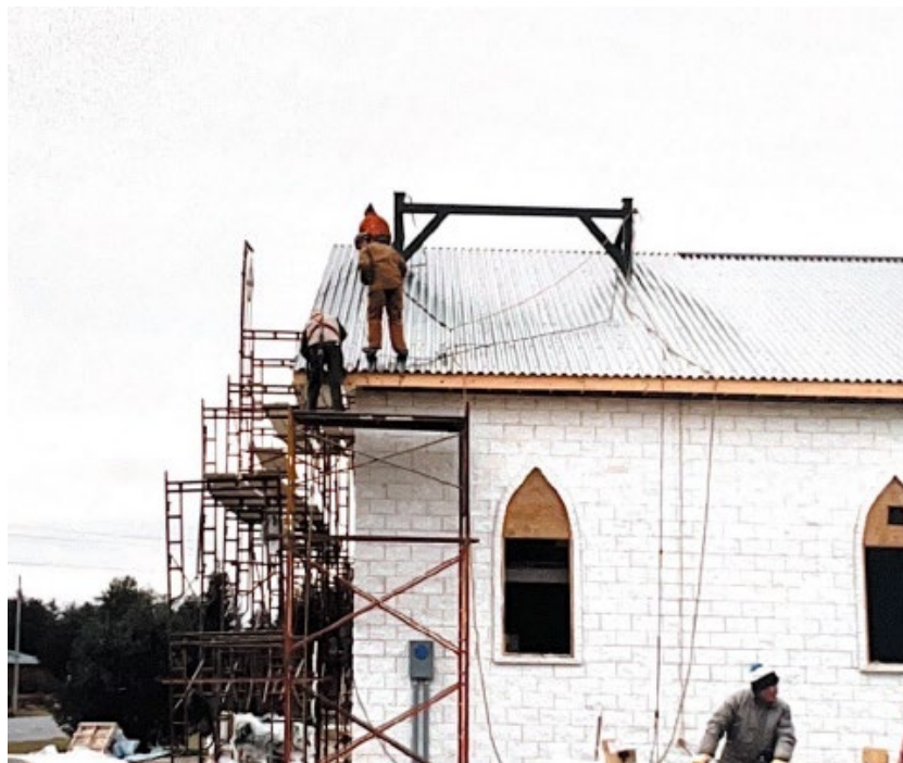
Figure 2 - Installation of metal roof (1998)
