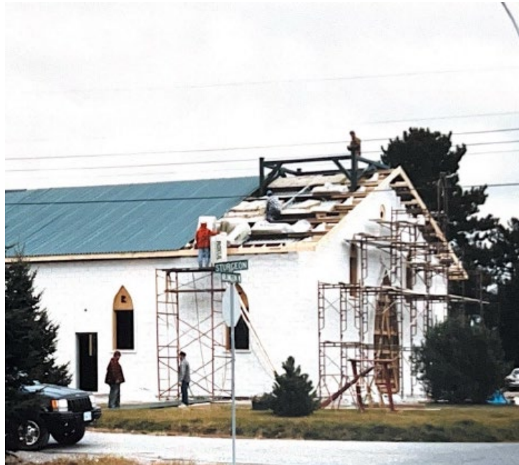
Figure 1 - Installation of metal roof (1998)
